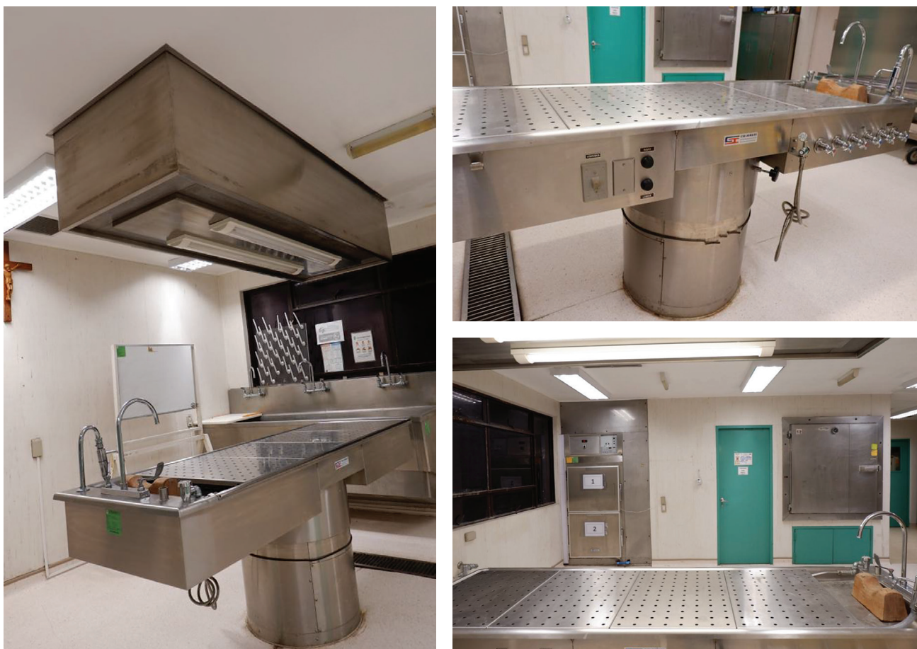
Figure 2. Autopsy table with down draft ventilation. The autopsy table is designed for dissection of cadavers and includes a recessed top which eliminates the need for a body tray. The downdraft system provides a safe environment, completely ventilating formalin vapors down and away from the user.
